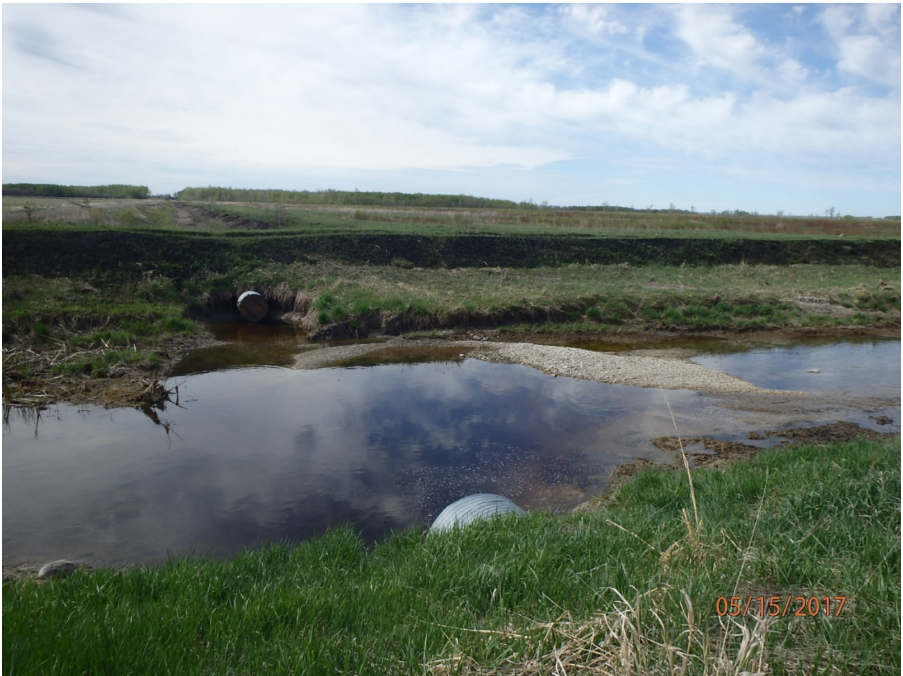
Outlet end of Huseby Pipe into SD 95 Lat 1 Ditch – looking south. Sediment buildup in Lat 1 to be removed.
